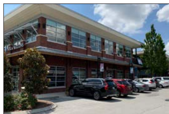
301 Manufacturer Road Northshore
